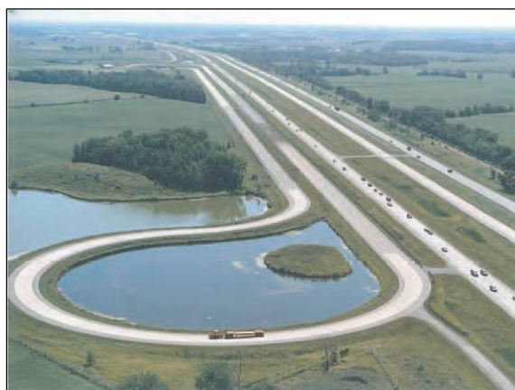
Figura N° 4: Ncat Pavement Test Track
