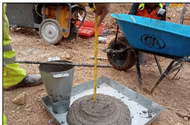
Figura 72. Slump de shotcrete GMO-003, 9 1/2"
